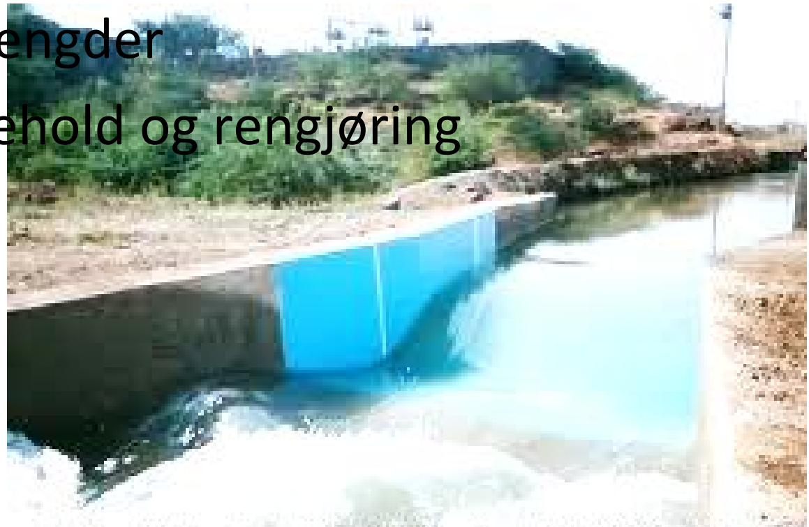
Parshall Flume Of 150 Cusecs Capacity With Digital Water Stage Recorder @ ch 5400 of Mangi Right Bank Canal Of Malgi Medium Project Tal Karmali Dist Solapur.
